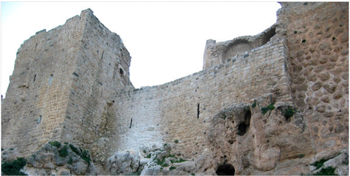
Photo 4. Masyaf was one of the most sufficiently fortified Assassin strongholds. Thick walls, far-projecting towers and numerous loopholes are among the defensive features that put it in one line with the strongest Crusader castles.
