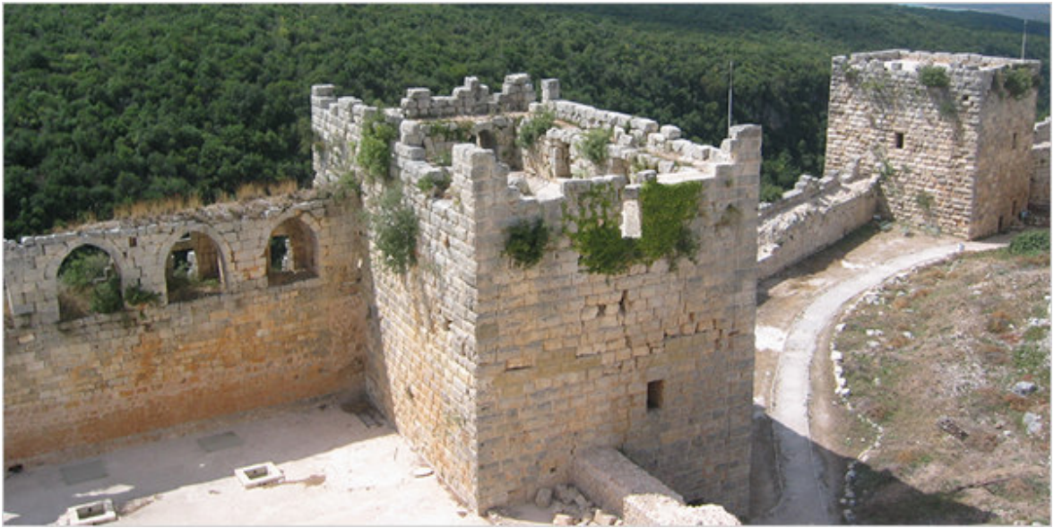
Photo 3. Saone, one of the finest examples of Crusader architecture, has nevertheless inherited a number of defensively weak Byzantine features.
